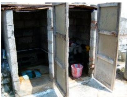
Toilet and Washing Area
